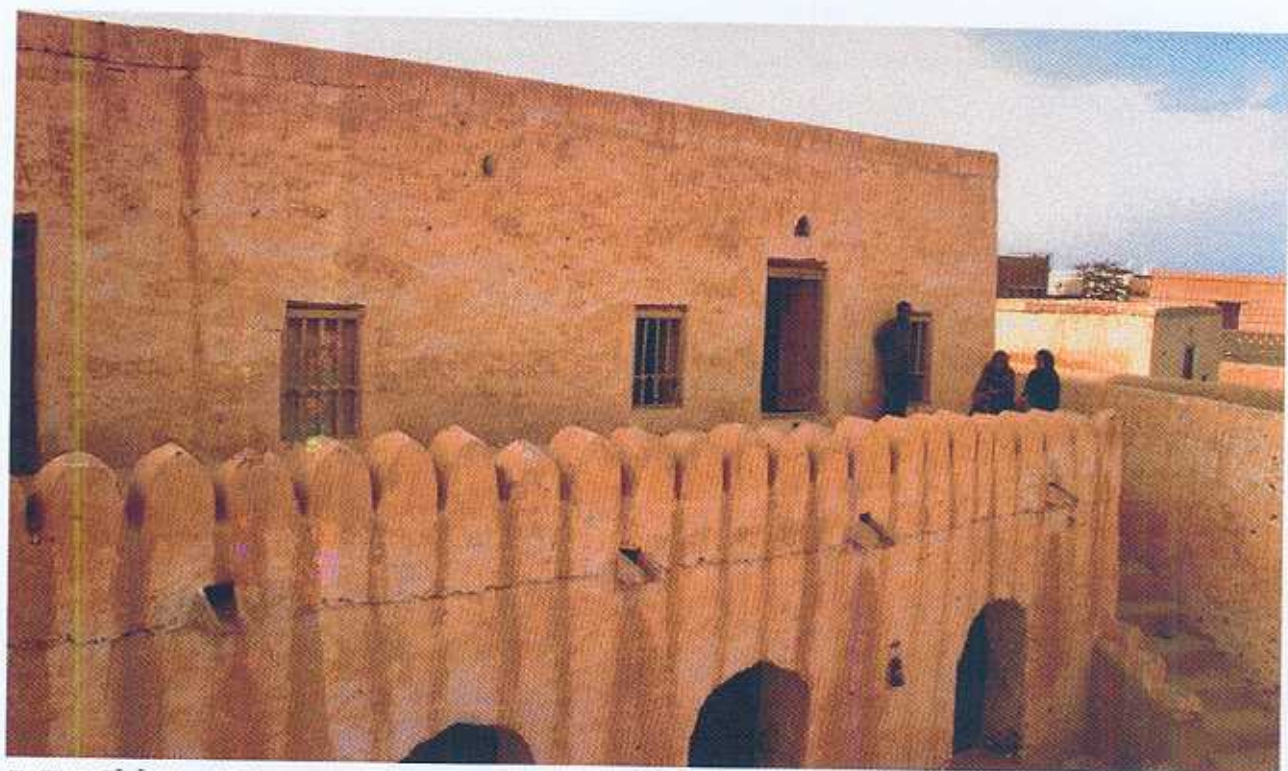
PLATE 17. Īwī, House VI. Courtyard view from S.
