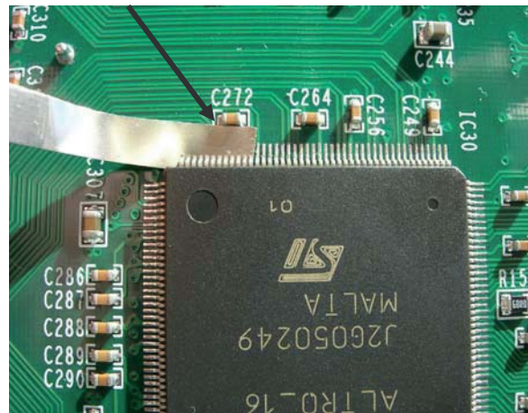
Fig. 5: Incompletely soldered pins (indicated by the strip inserted) of one of the ALTRO chips.
